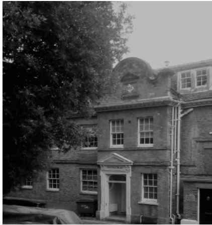
Front Elevation on Hillside Street
