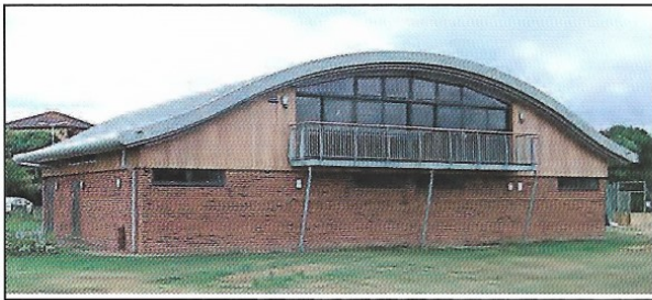
South Road Sports Hall
