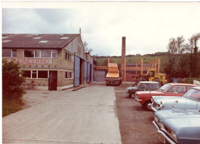
Hythe Engineering Factory C under construction 1970 approx.
