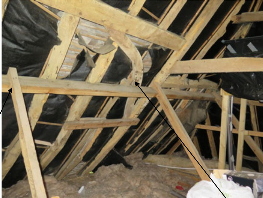
Newer purlins with diagonal braces to tie beam
