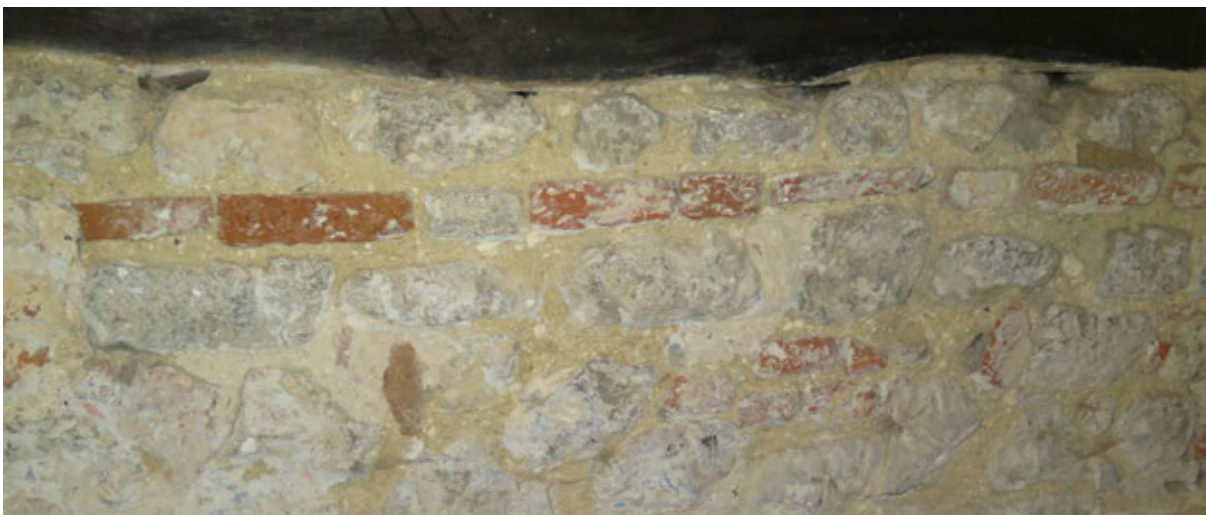
Part of inner wall showing Roman style bricks
