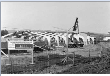
The Former Seaboard Offices Military Road, 1976/77
