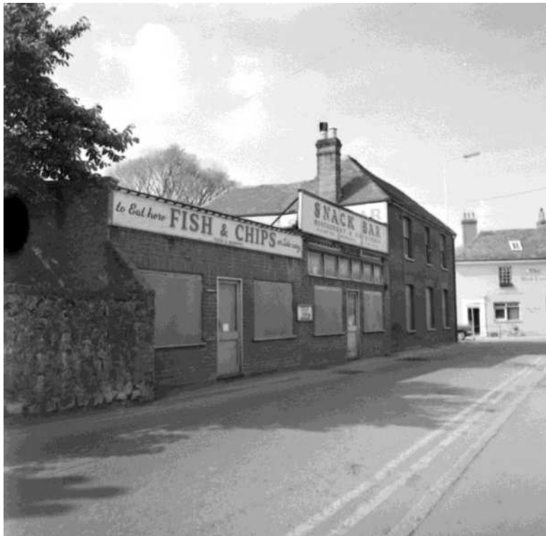
Above: The Snack Bar, Rampart Road shortly before demolition in 1971 – photograph by Jack Adams
